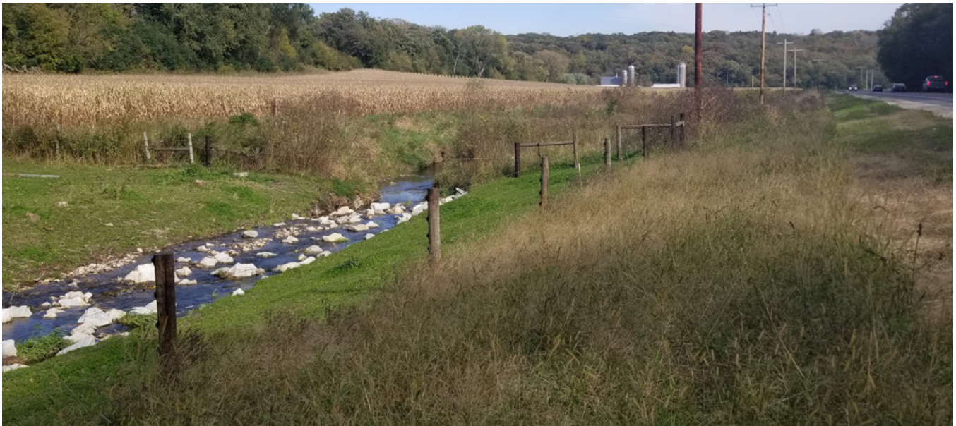
A naturalized, riprapped embankment between a trout stream and TH52 north of Chatfield, MN
