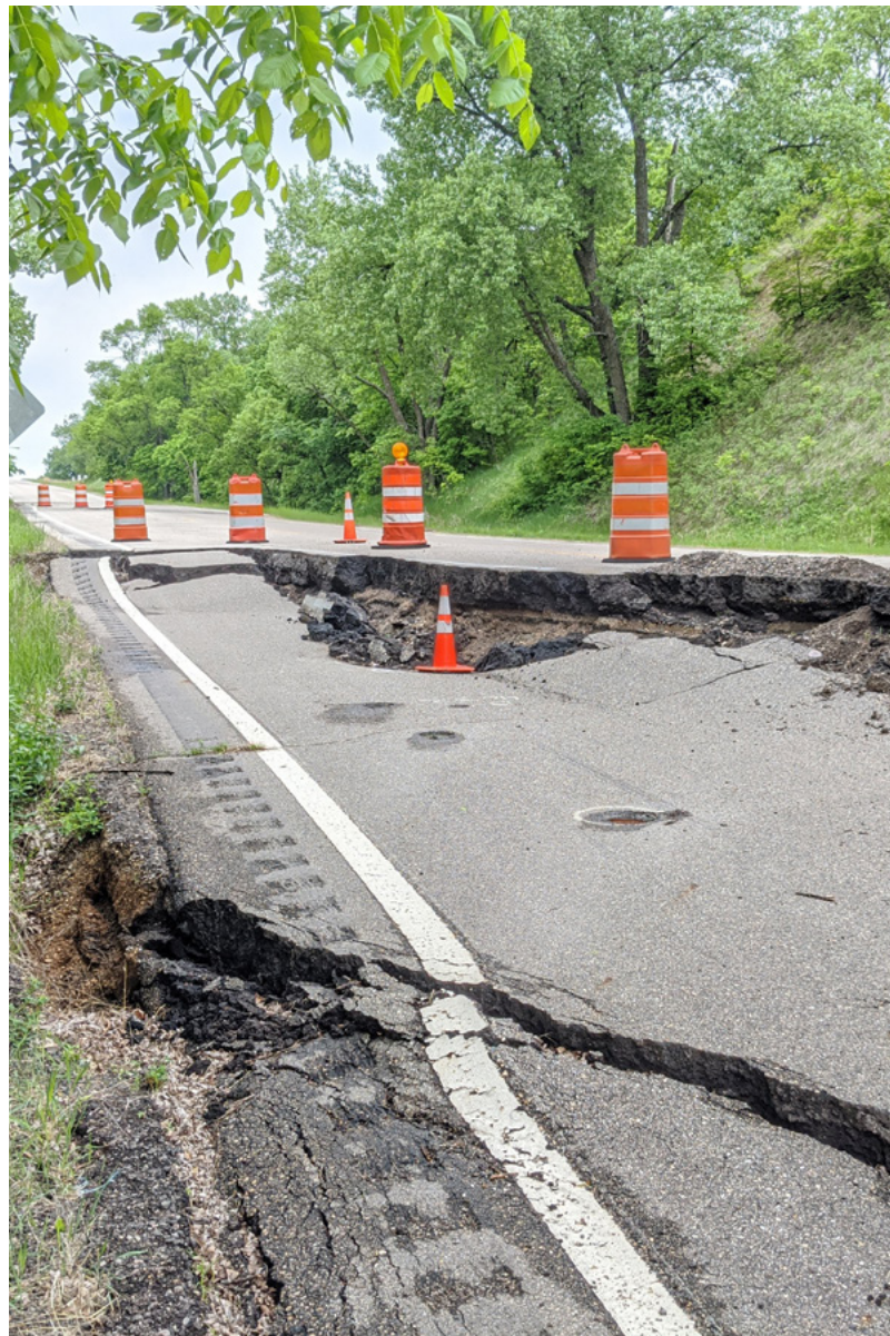
A springtime landslide permanently closes a section of Hwy 67 along the Minnesota River valley.
