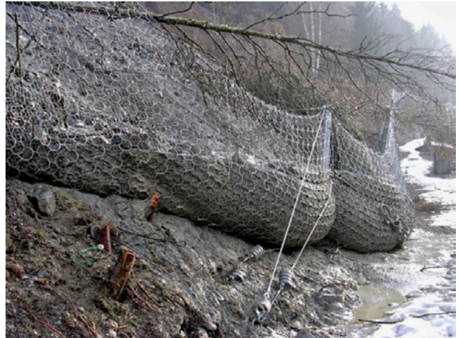
Example of debris flow detention fencing holding back debris flow.
